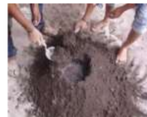
Fig 5 Mixing with concrete
